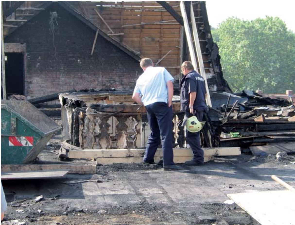
Duchess Amalia Library, Weimar, Germany: upper level damage following fire (Photo: P Rohlén)
