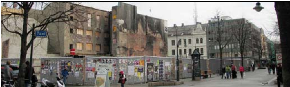
Trondheim, Norway following the December 2002 fire.
